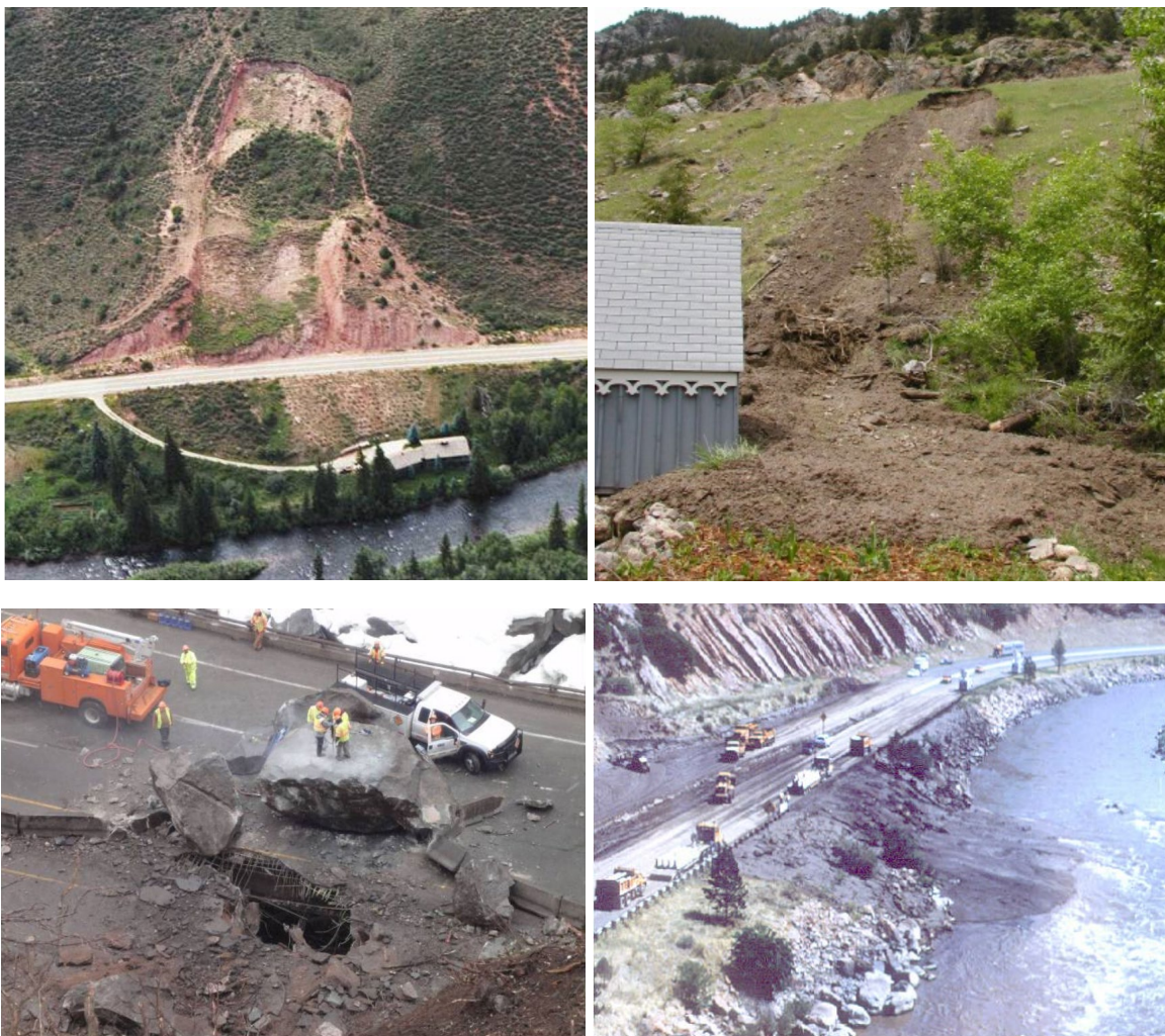
Figure 2-1. Examples of the landslide geohazard types considered for this study: deep landslide (top left, photo by CDOT), shallow landslide in an embankment (top right, photo by CDOT), rockfall (bottom left, photo by CDOT), debris flow (bottom right, photo by USGS)
